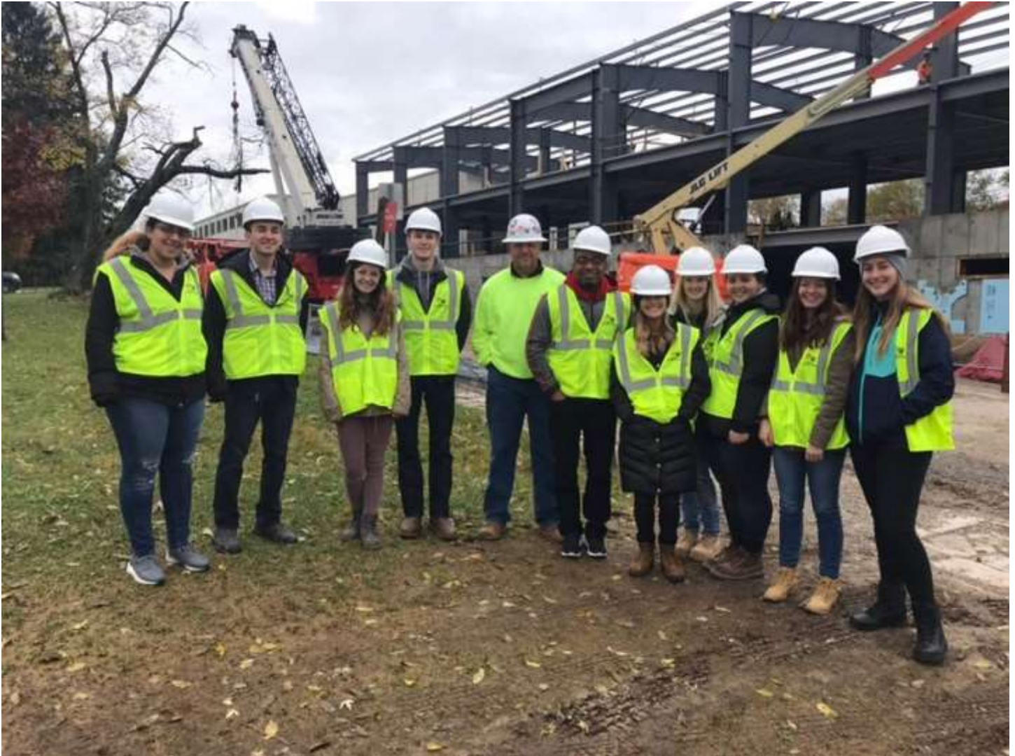
Students attend tour of IU Fines Arts Building and Ballantine Hall construction projects. Thanks Gino!
